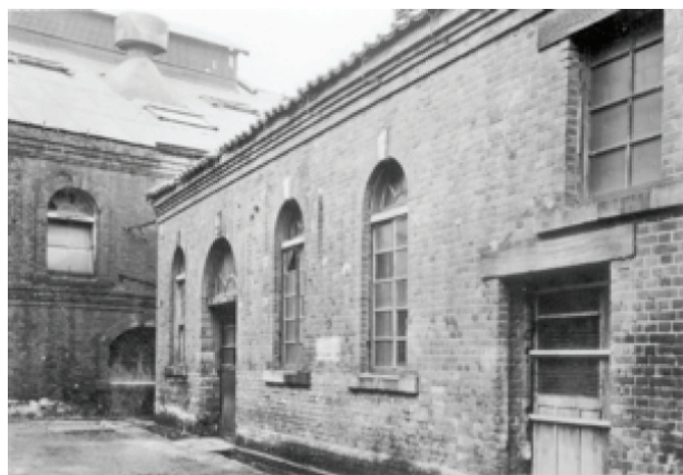
Figure 3. Glasshouse buildings photographed in 1962, just before demolition. The flint glasshouse is the left of the two buildings. In 1877 it had a chimney which was 24 m in height, with a diameter of 6.6 m at the base and 2.42 m at the top. (This chimney is visible in the full photograph in Figure 2.) The ventilation on the roofs here may be a 20th century addition. Reprinted by courtesy of Meijimura Museum
